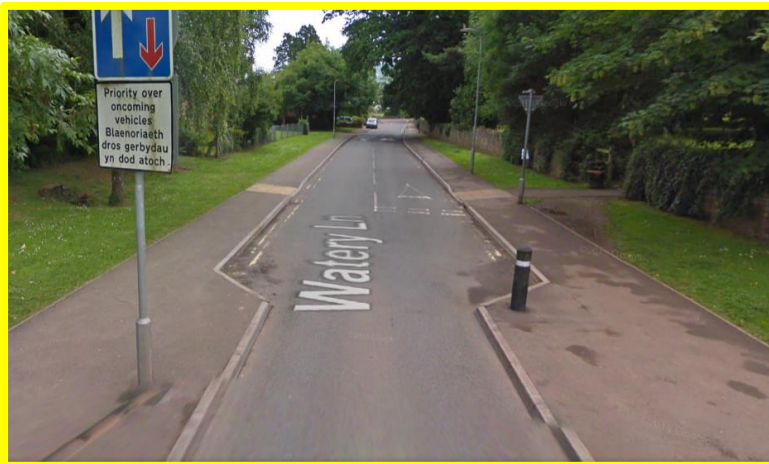
View eastwards along Watery lane (towards Rockfield Road). The image shows adopted public footway to both sides of the highway, along with traffic calming measures and drop kerbs with tactile paving.
